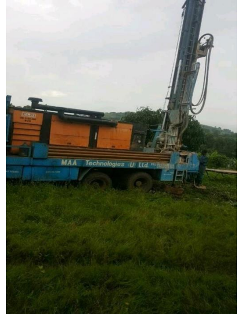
Drilling of the borehole by MAA Technologies in Kashangura and Nsasi Villages.
